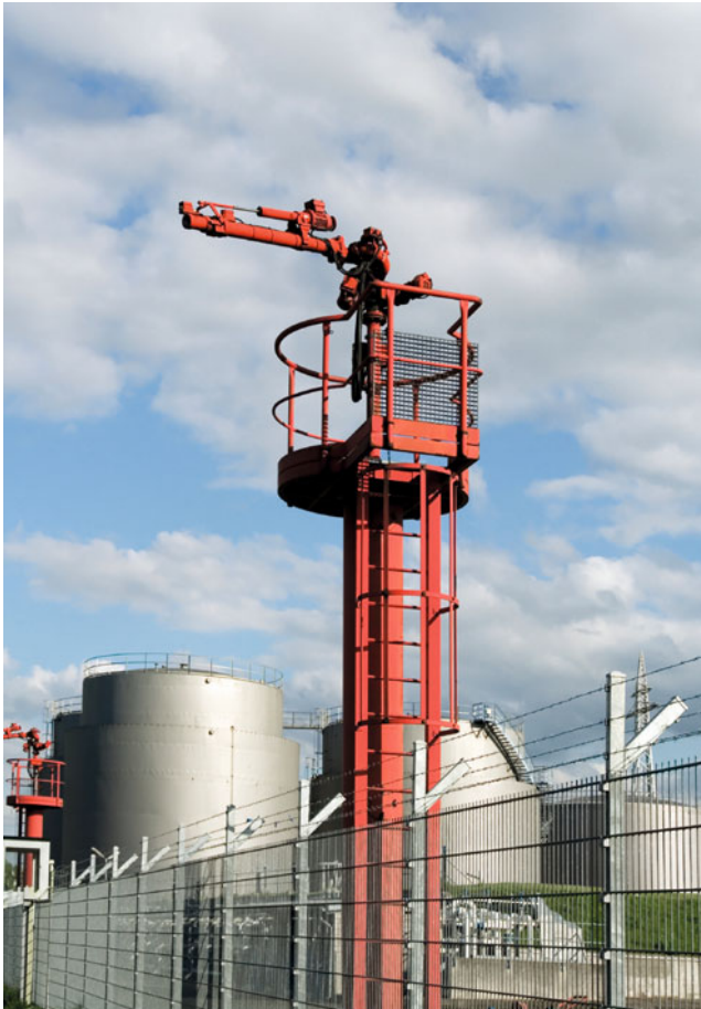
Figure 17.13 Fixed point fire-fighting cannon Source: iStock.
