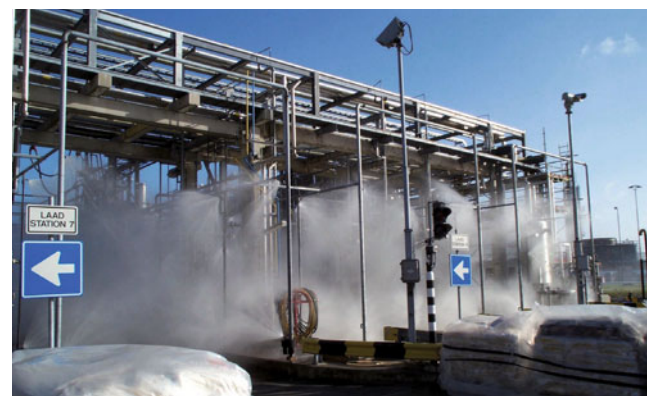
Figure 17.3 Fire deluge system Source: Frontline Fire International.
