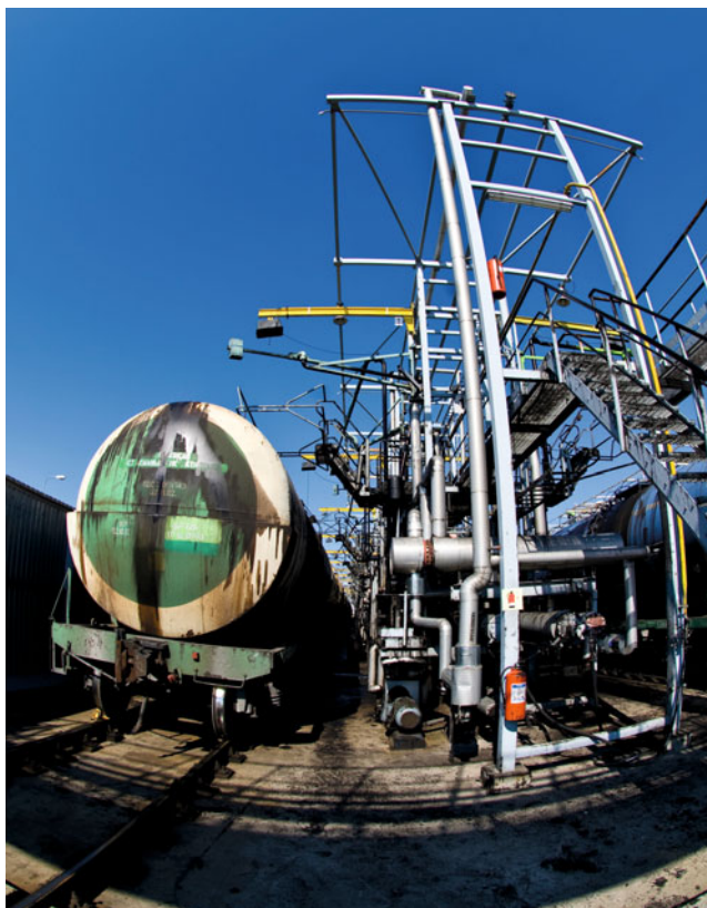
Figure 20.6 Loading arrangements for rail tankers Source: Dreamstime.
