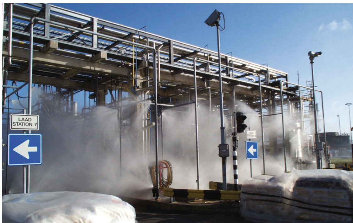
Figure 9.2 Fire deluge system
