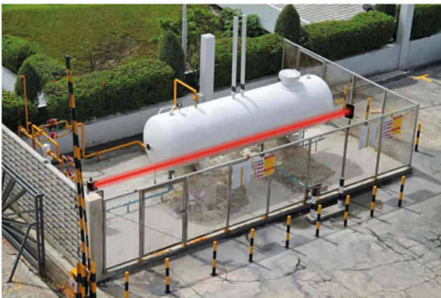
Figure 17.2 Infrared beam detector in situ Source: Dreamstime.
