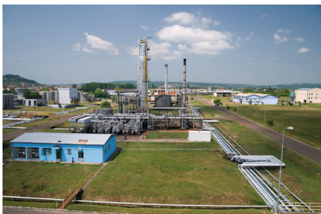
Figure 11.5 U-shaped configuration in pipework Source: iStock.
