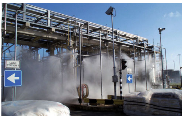
Figure 13.2 Fire deluge system Source: Frontline Fire International.
